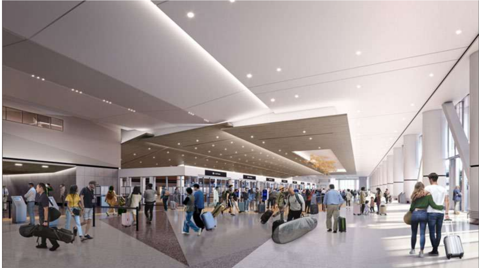
Figure 5 | New T1 Ticket Lobby
