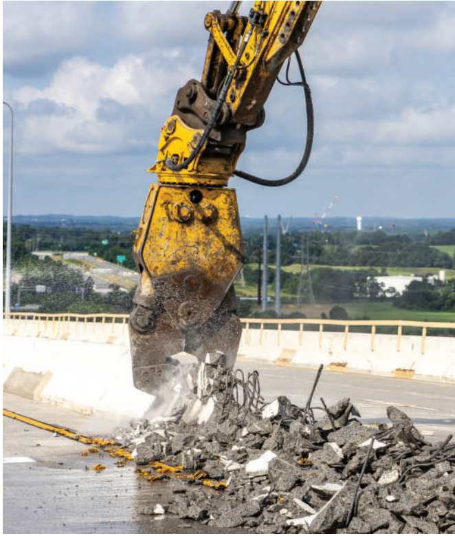
Key Bridge Demolition - Deck Removal
